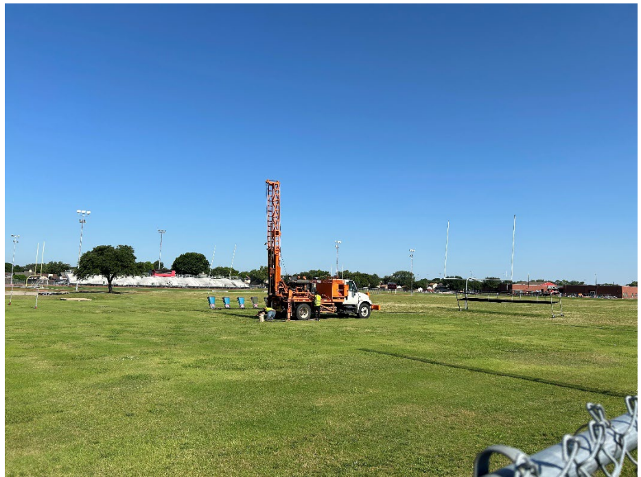
North Garland GeoTech drilling
