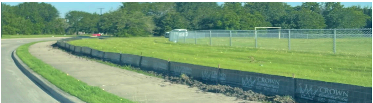
SW3P fencing installed at Centerville for bus lane construction.
