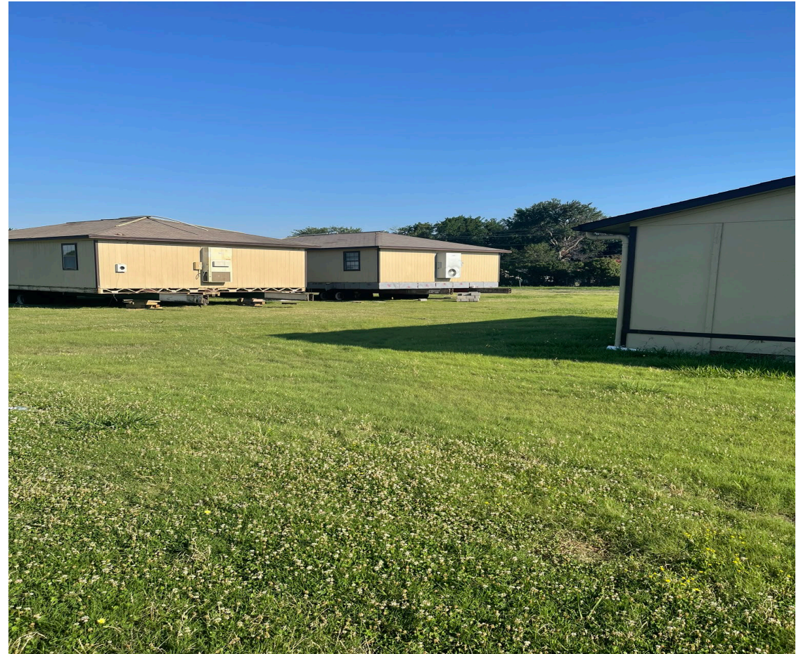
Portable Relocation to Centerville Elementary
