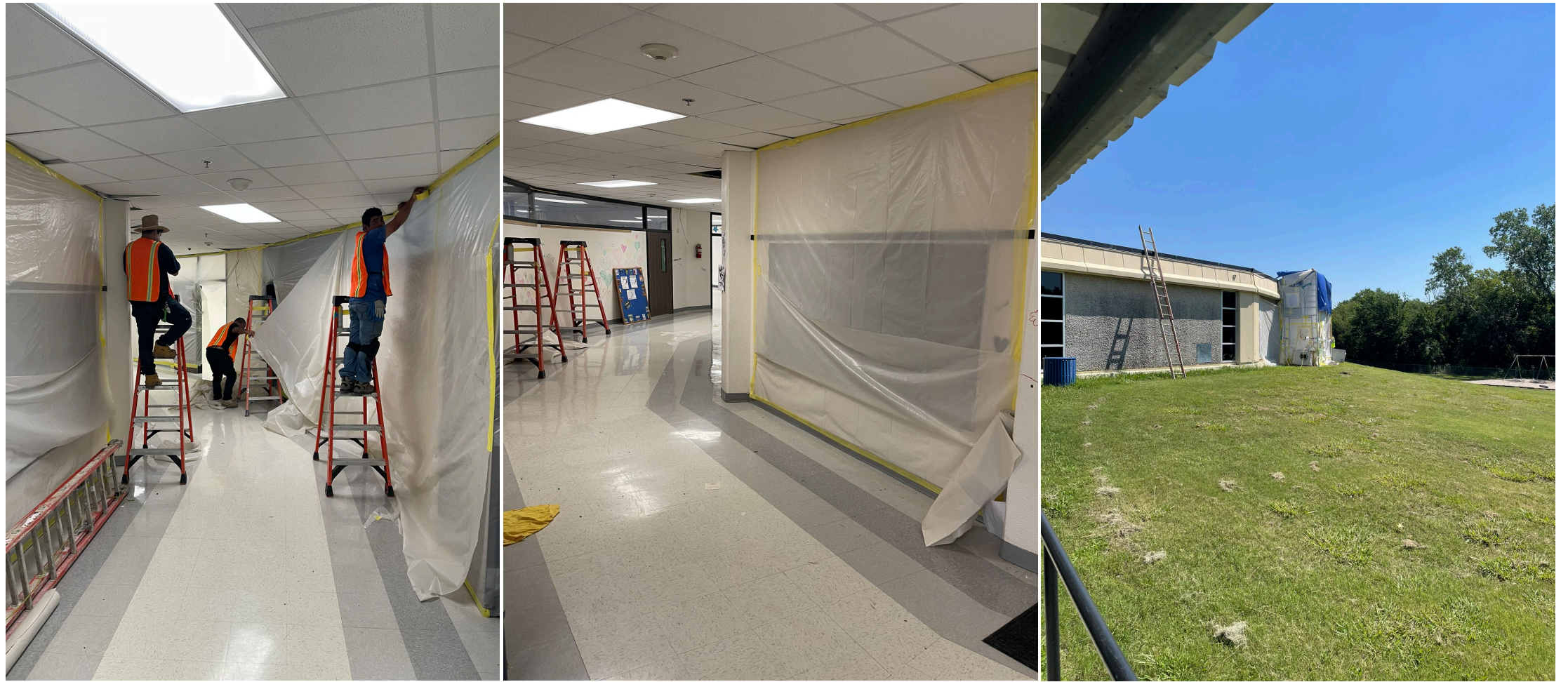
Interior / Exterior Abatement
