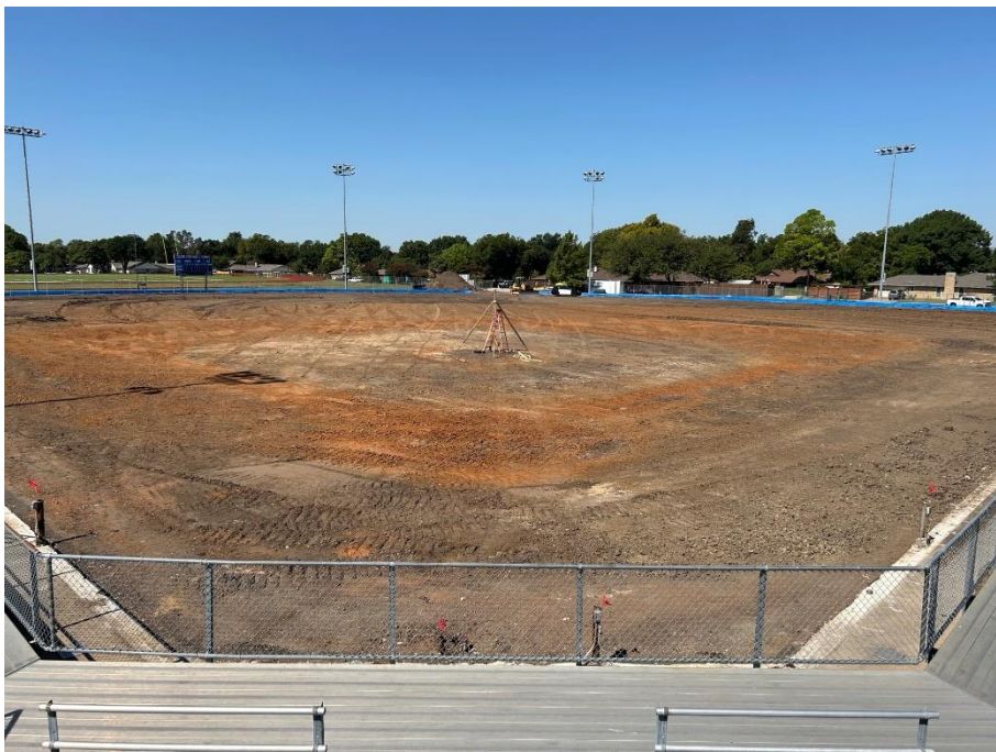
South Garland, Final grading for Baseball Field
