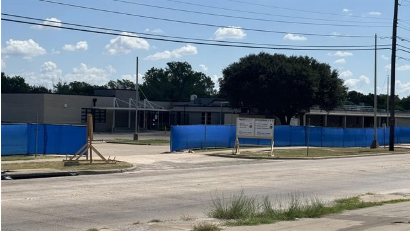
Lee Lewis Construction Signage and Fencing
