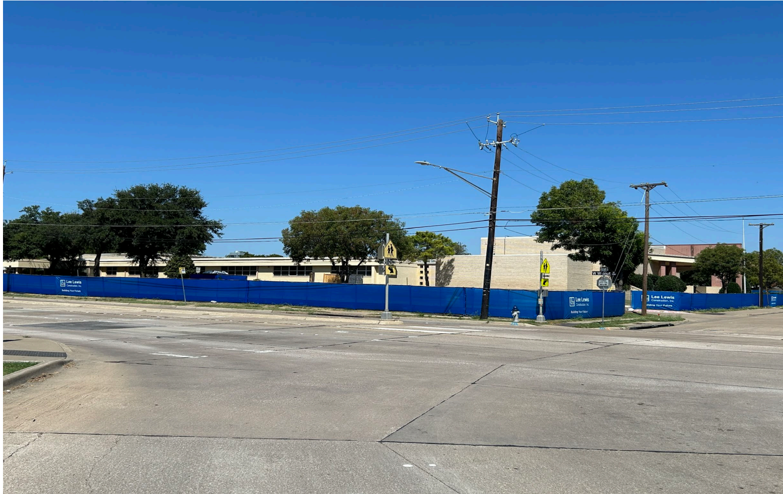
Lee Lewis Construction Signage and Fencing
