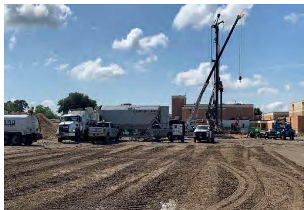
South Garland: Progress
