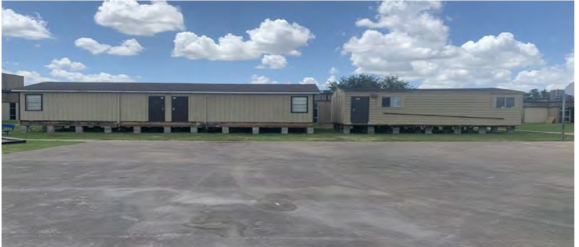
Heather Glen Elementary Portable Relocation
