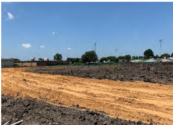
North Garland: Progress
