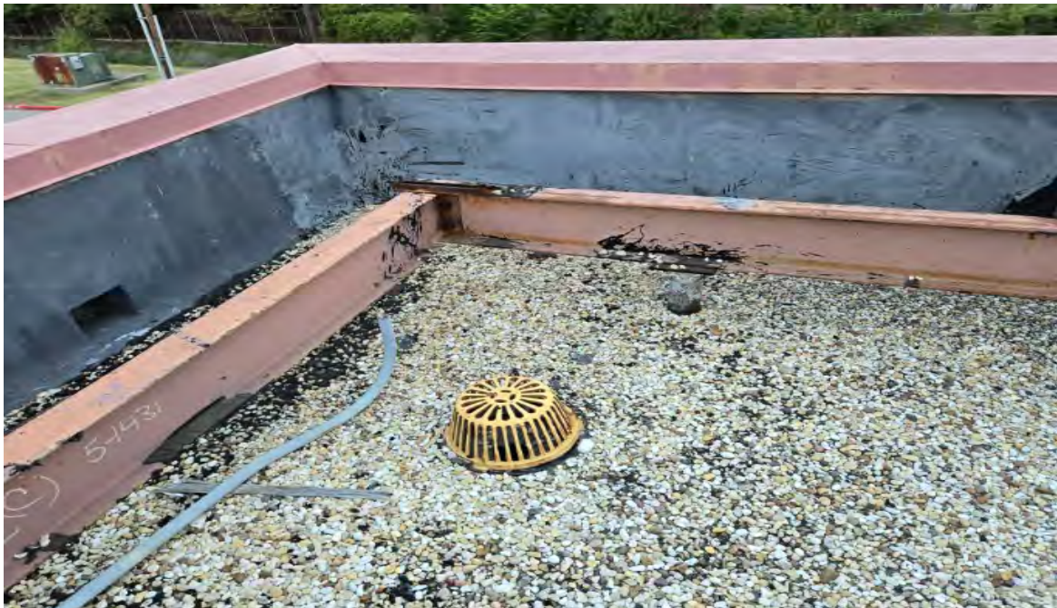
Old gravel will be removed and any pipes will be raised and lifted off the new roof system.
